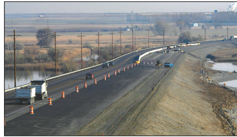
Construction progress at Casey Pond on new four-lane section near Burbank
