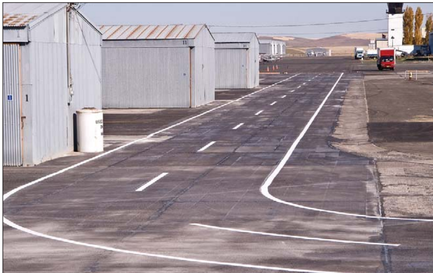
PHOTO: Airport's South Aviation Ramp improvements included diamond grinding, concrete panel repair and replacements, installation of an enhanced storm water drainage system, surface seal coat and striping.
