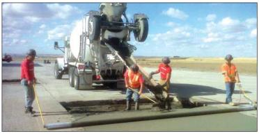
PHOTO: Construction crew pours new North Ramp concrete. Port file photo.
