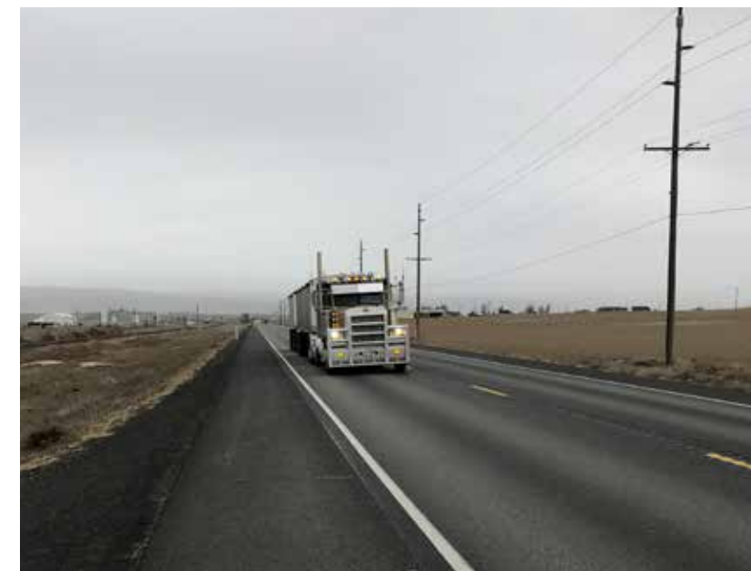
Central and Eastern Washington's economy relies on the ability to move freight. Four-laning US 12 improves freight mobility and safety for travelers using the corridor.
