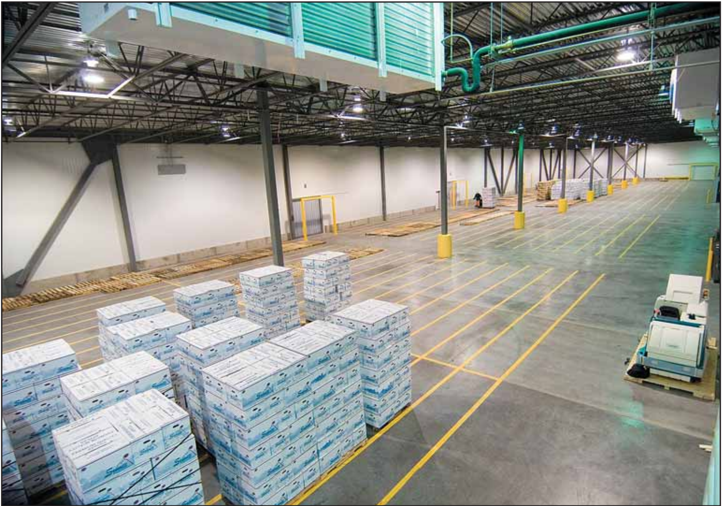
A part of the whole...this view is of less than half of Railex's 200,000 square foot transloading center at Wallula. Overall the structure is five football fields long, 140-foot wide, with controlled storage kept at temperatures as low as 33-degrees. Fresh produce stored here is loaded into specially-designed refrigerated rail cars that make up the produce train destined for direct travel to a similar facility in New York for distribution to East Coast markets.
