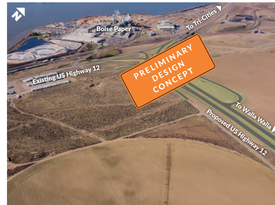
Proposed US Highway 12, looking west to the Boise Paper Wallula Mill and the proposed US Highway 12 intersection.
