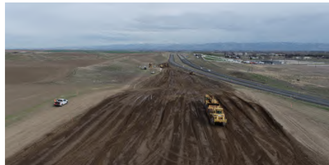
WSDOT and contractor crews break ground on the project in March 2021.
